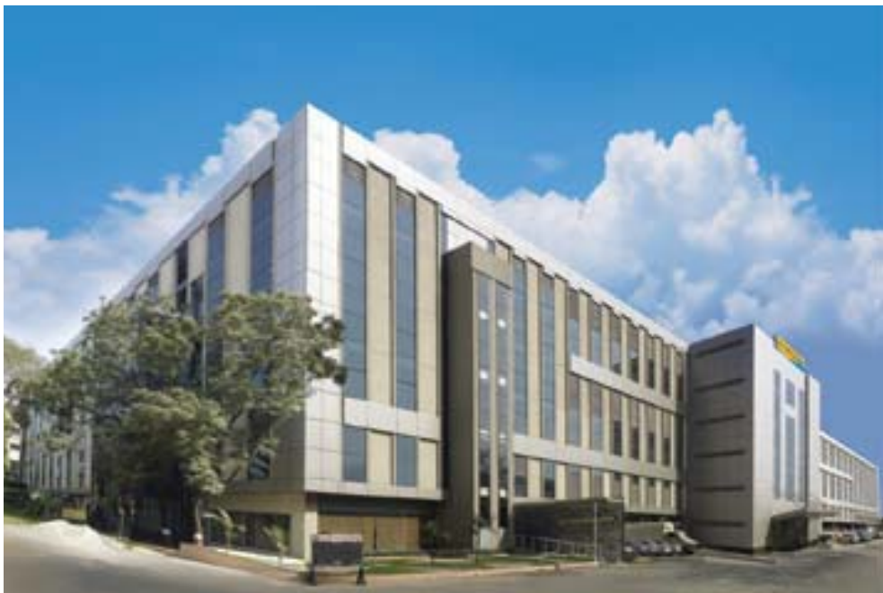
Powai Switchgear Factory, Mumbai.
